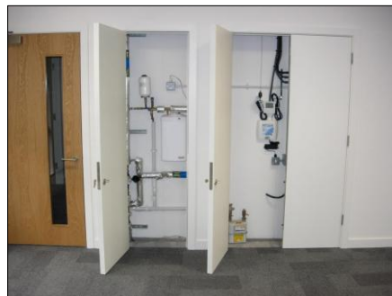
PHOTOGRAPH 8 TYPICAL RISER CUPBOARD (BUILDING 4)
