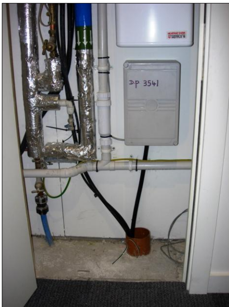
PHOTOGRAPH 7 TYPICAL RISER CUPBOARD AND BT ENTRY (BUILDING 4)
