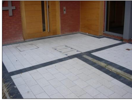
PHOTOGRAPH 5 BT CHAMBER OUTSIDE BUILDING 4
