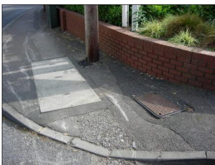
PHOTOGRAPH 1 BT AND VIRGIN MEDIA CHAMBER AT ENTRANCE ON GARDNER ROAD (EAST SIDE)
